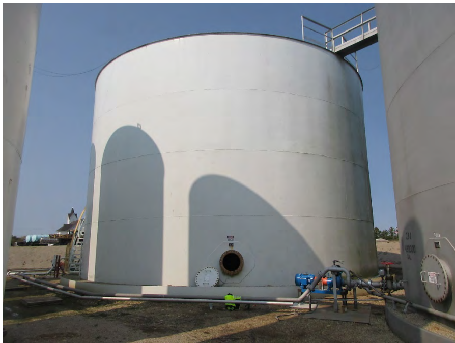
Tank # 1 51' Diameter x 32' High Tank Carbon Steel Construction 28% Nitrogen Solution
